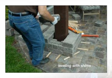
Leveling adjustments can be made by shimming with thin pieces of wood, ceramic tile wedges, or other devices to hold the first course level until the adhesive sets up.
