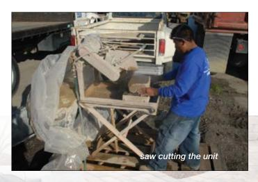
Cutting can be done with a masonry saw or by using a guillotine-type block and stone splitter. Saw cuts are more precise, will guillotine splits are faster.
